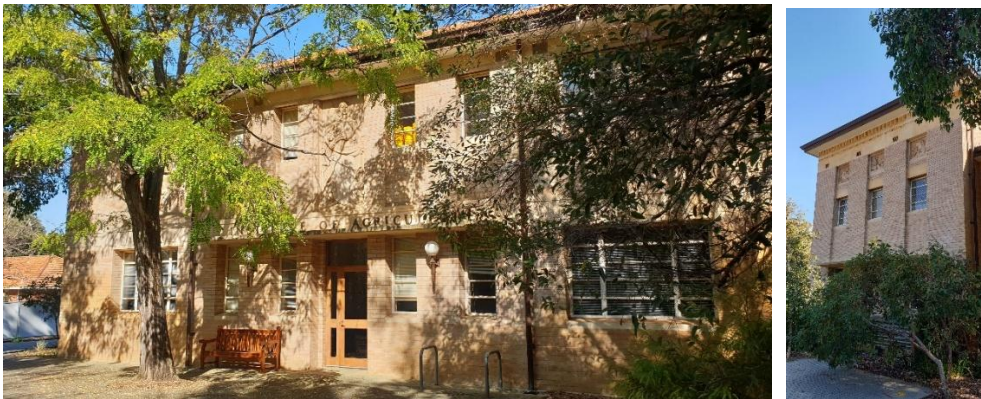
Baxter Cox & Leighton 1938 Department of Agriculture at UWA - north and east elevations (John Taylor 2019; see 'Crawley Campus', p.51 for drawing).
